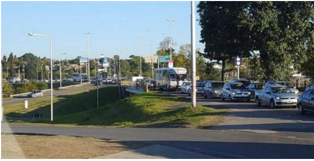
Fig. 6. Pre-toll route leading to subfluvial tunnel entry point.
