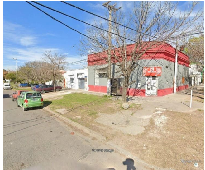
Fig. 3. Electromechanical workshop at the intersection of Ejercito Avenue and Gutierrez Street.
