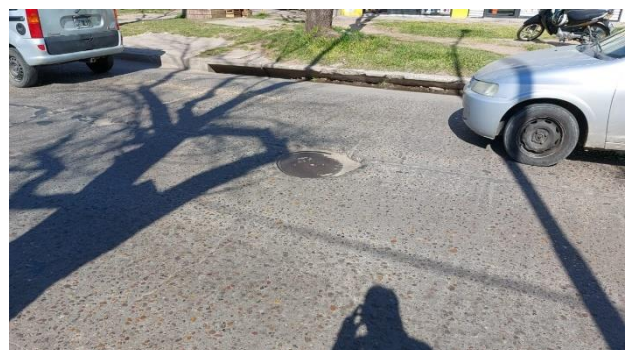
Fig. 13. Storm drain in Gutierrez Street.
