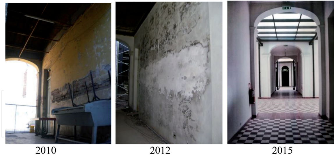
Figure 6. Evolution of the mortar compatibility process during rehabilitation of school building [2].
