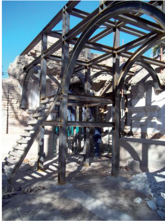
Figure 13. Support structure of masonry blocks, Saint Francis Ruins, 2011.
