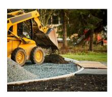
Once the stage 1 be ready, I am going to make the necessary land corrections to reach the work level. Then I am going to cover the land with a geotextile and on it we are going to place the gravel by using a mini loader.
