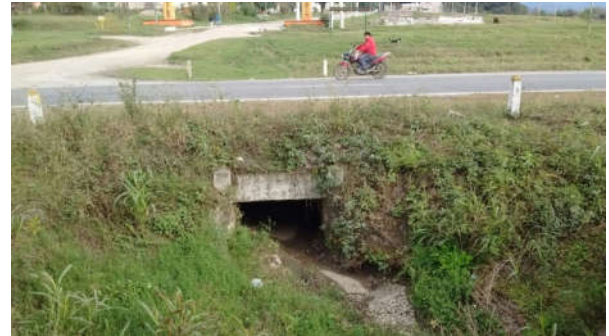
Figura 11: Alcantarilla Ruta 9, km1309
